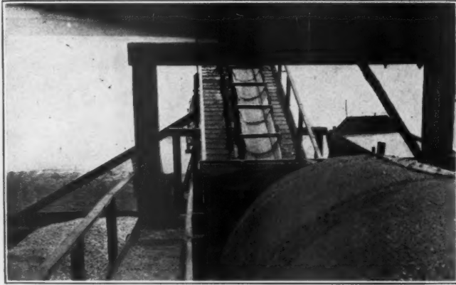
Sizing Screen and Conveyor for Loading Barges
